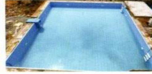
Liner Renovated Pool with PLF at HYDERABAD
