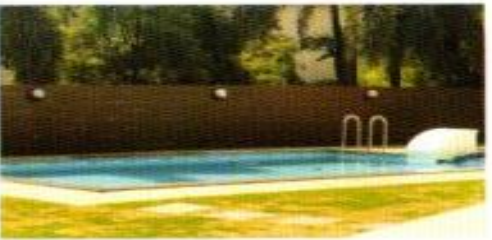
Deck Mounted Prefab Pool at LONAVALA
