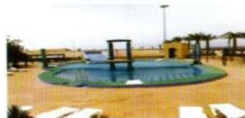
Pipeless Filter in JORDAN
